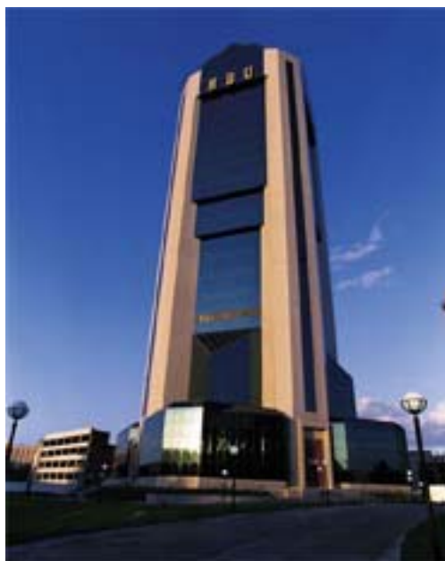
National Bank of Uzbekistan
